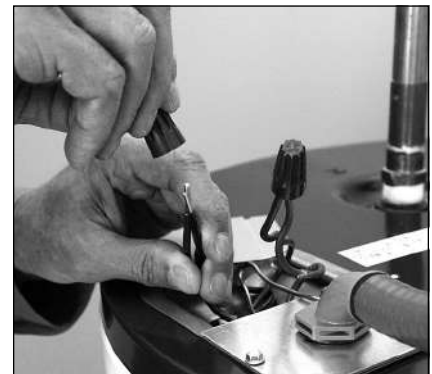
Figure 19 - Connecting the electrical wires.
