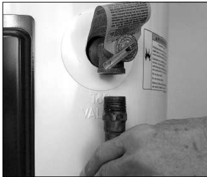
Figure 11 - Removing the T&P Relief Valve discharge pipe.
