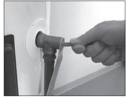
Figure 38 - T&P Relief Valve
