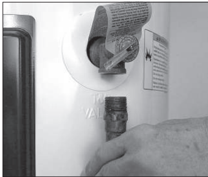
Figure 11 - Removing the T&P Relief Valve discharge pipe.
